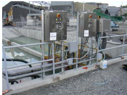
Wheel Wash Systems Control Panels UL & CSA Certifications, MobyDos Flocculent Pump for Rapid Solids Settlement
