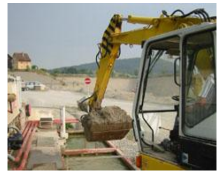
Emptying the Recycling Tank with an excavator
