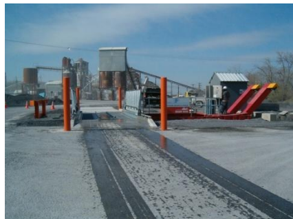
Moby tank recycling system 20.000 Gallons, automatic solids removal, flocculent systems, safety railing, water cannon wash.
