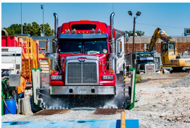
MobyDick Wheel Washing at the Ahrens Site
