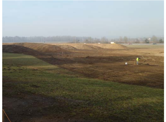
Image 2: Humus deposit on the building site.
