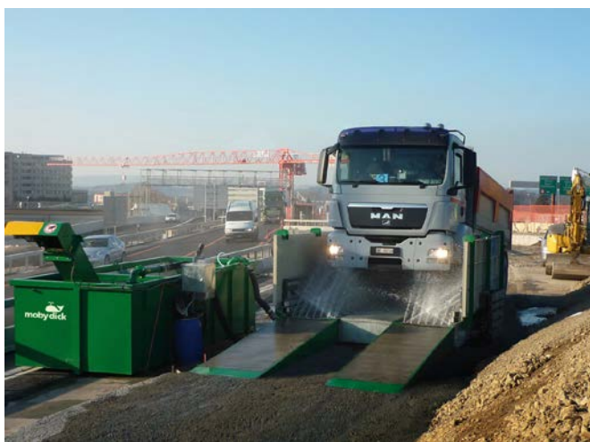
Figure 1: MobyDick ConLine Mobile on T2 motorway bridge structure
